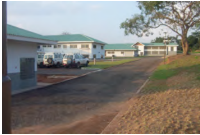
Main building Cafeteria Workshop Guesthouse with eight appartements
